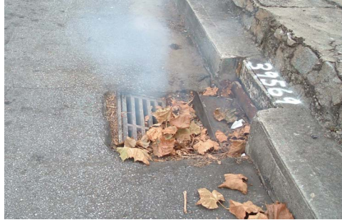
Smoke rises from a storm drain during smoke testing in the McDaniel Basin.
