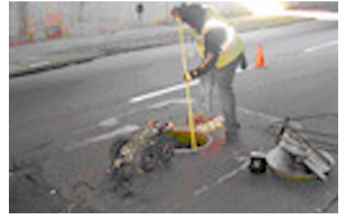
Field crew member prepares manhole for CCTV inspection on Peters Street.
