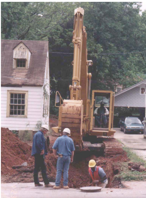
Open-cut construction on private property.
